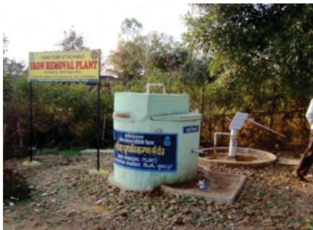
Figure 55: NEERI Hand Pump Attachable Iron Removal Plant
