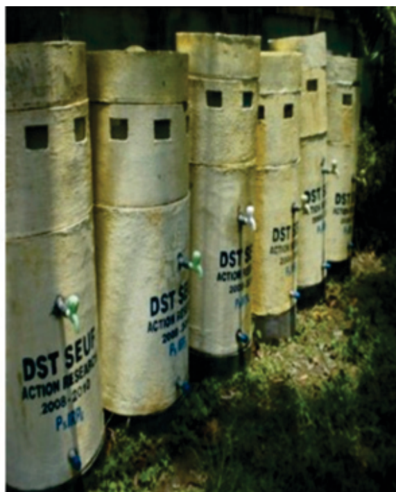
Figure 59: SEUF Iron Removal Plant (IRP)
