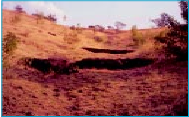
Gully Plugging on hill slopes
