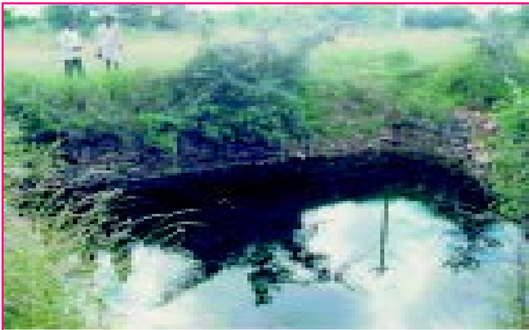
RECHARGING WELL UNDER IWDP PROJECT
