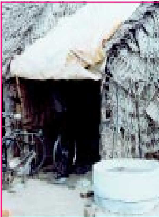
Thatched roof covered with a gunny bag In a cycle shop
