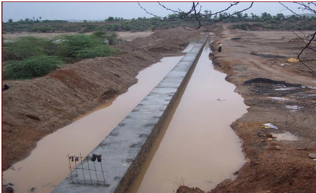
8.30 c A completed Sub Surface Dyke
