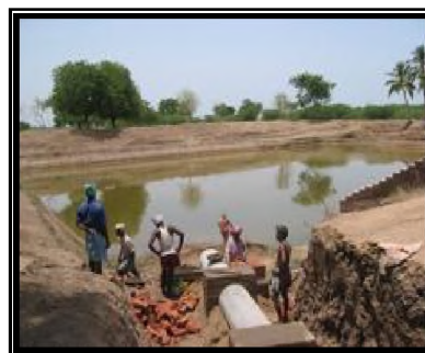
8.19 (c) Supply Channel
